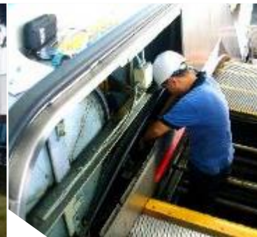
On-site Assembly & Maintenance
